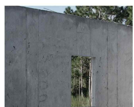
Poured in Place Concrete
